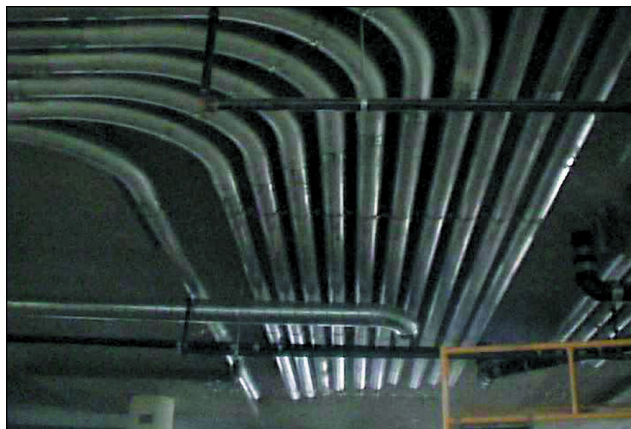
Figure 2 — The Ford Field project incorporates the latest BeverageCHASE™ Systems technology. Components are available in a wide variety of sizes and degree of bend to accommodate most needs. Custom bends are also available.
