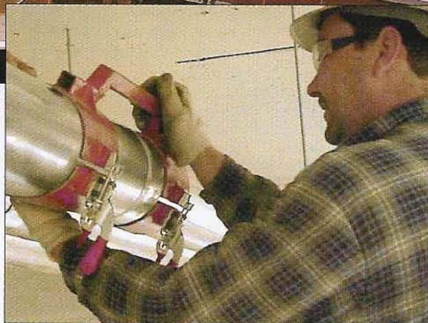
Colombo Sales and Engineering developed an alignment tool that allows beverage chase systems to be precisely connected in the field with 3M VHB Double-Coated Foam Tape.
